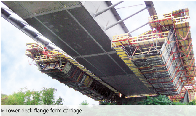
► Lower deck flange form carriage
