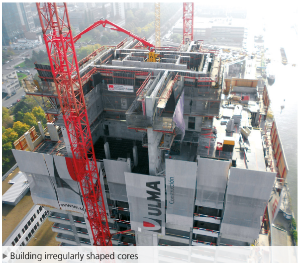
► Building irregularly shaped cores
