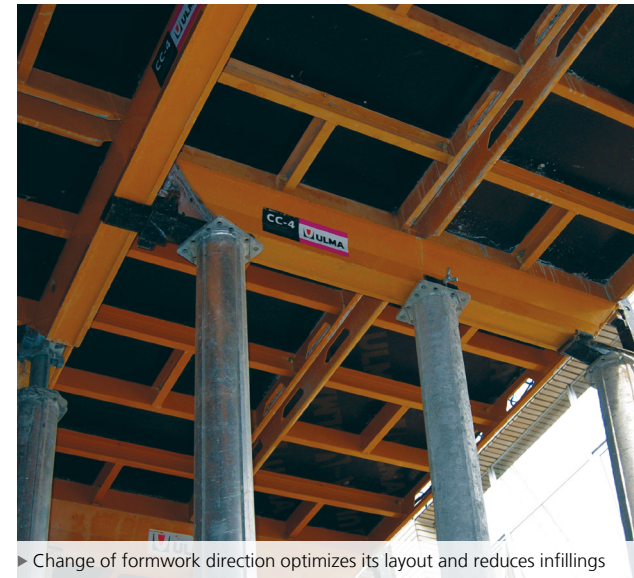
► CC-4 panel system supported by ALUPROP towers
