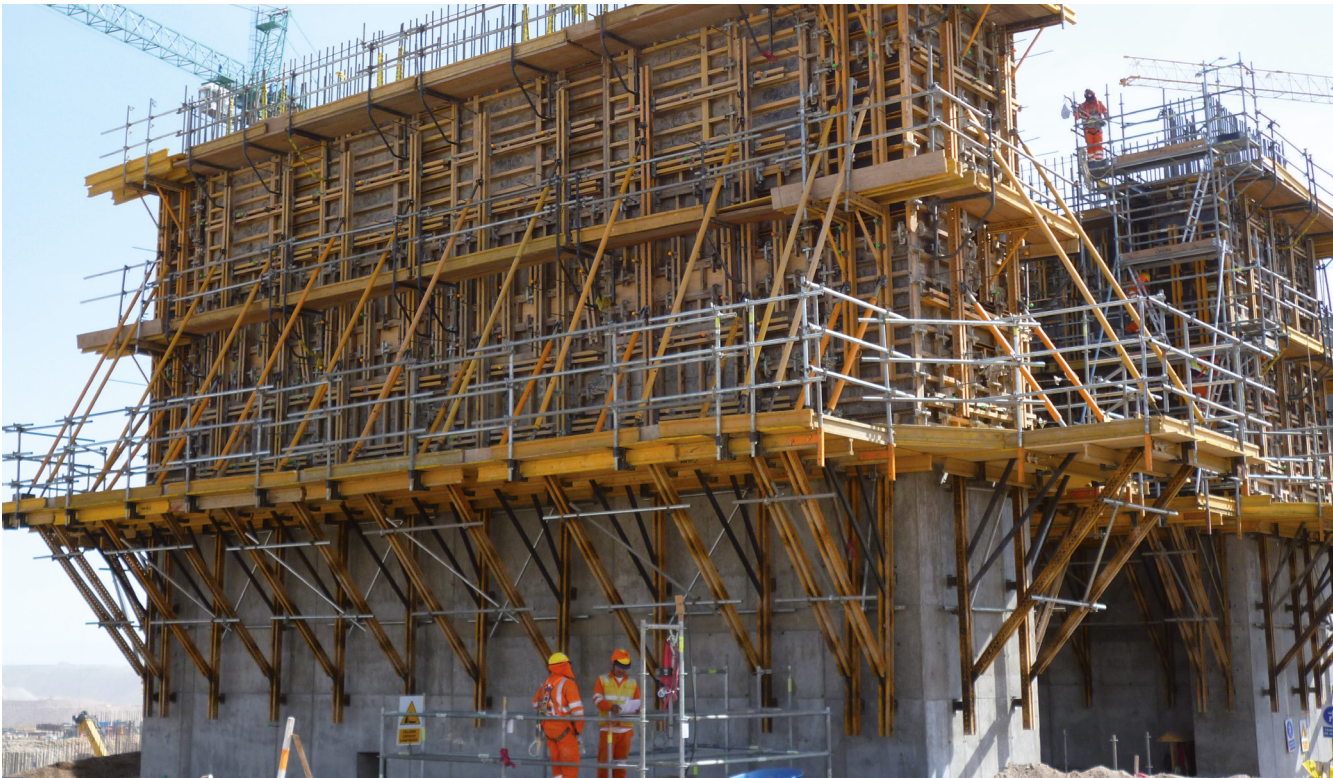
Crane assisted climbing brackets with available platforms for added safety and cone recovery.
