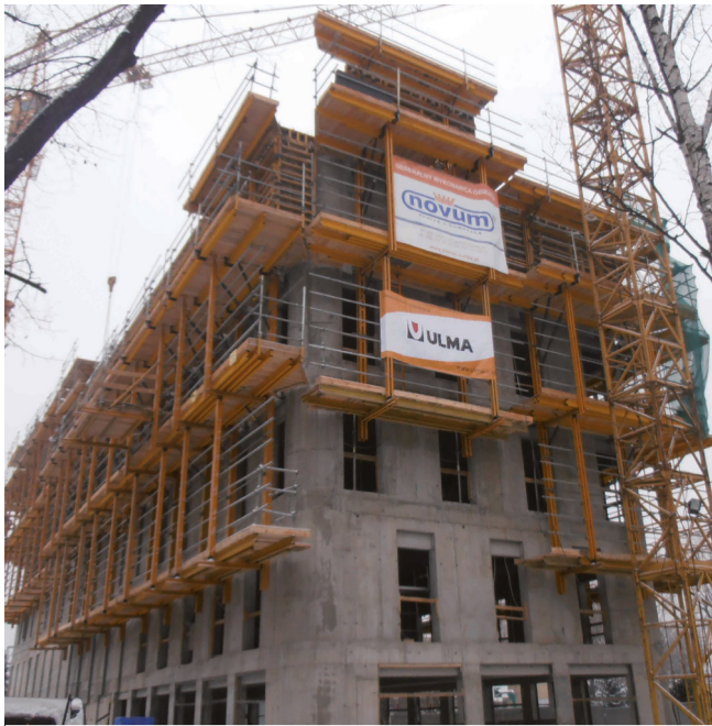
► Hydraulic movement allows for quick and easy forming
