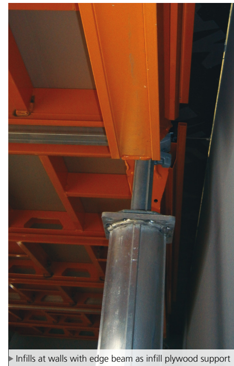
► Change of formwork direction optimizes its layout and reduces infillings
