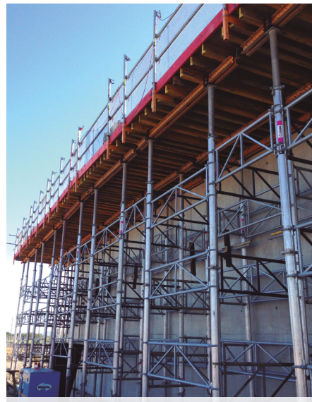
► Bracing between ALUPROP props and towers using tube and clamps and/or with bracing frames
