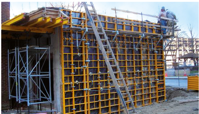
► Attachable safety brackets for work at multiple heights
