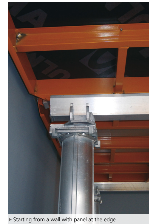
► CC-4 panel system supported by ALUPROP towers
