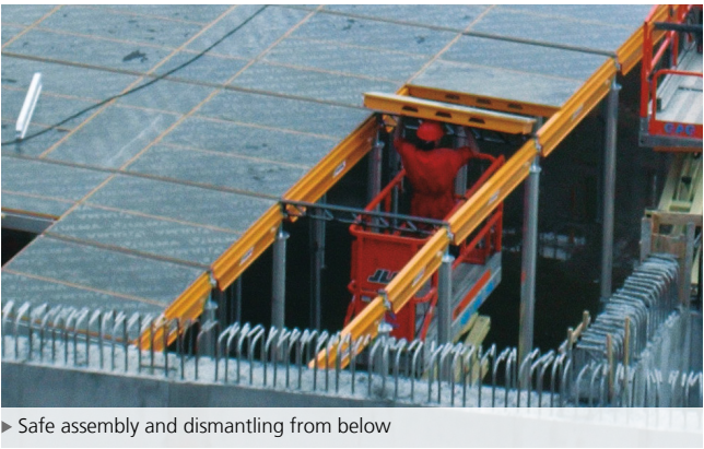
► Safe assembly and dismantling from below
