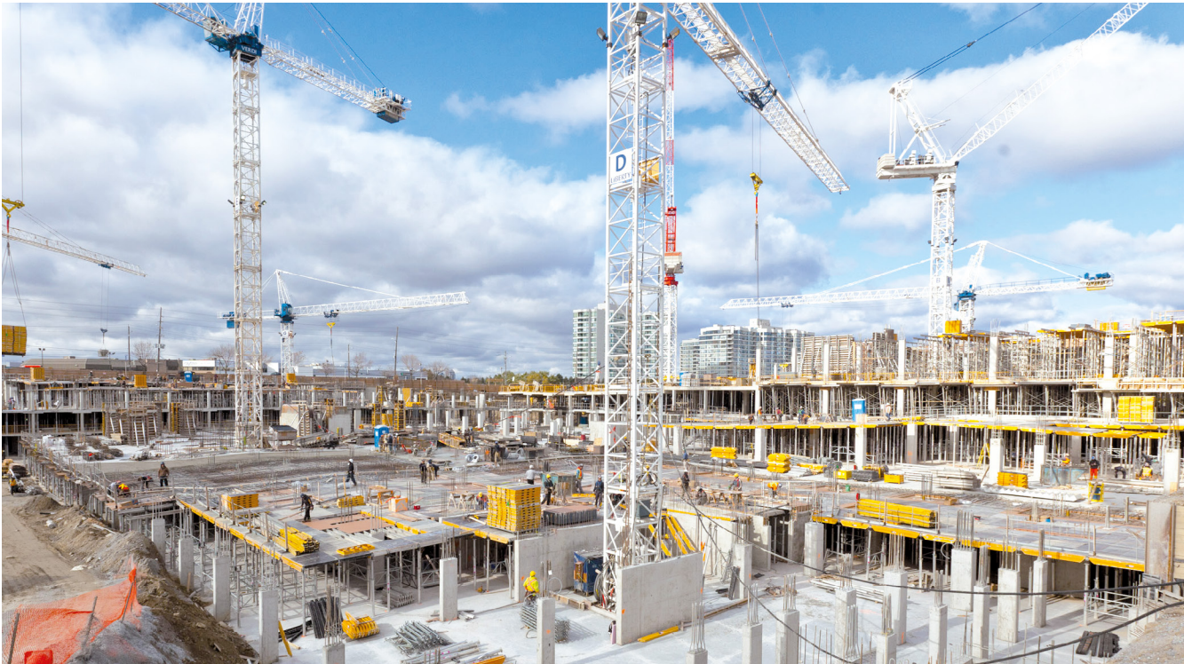
Light, safe panelized drop head shoring system with high productivity and excellent concrete finish.
