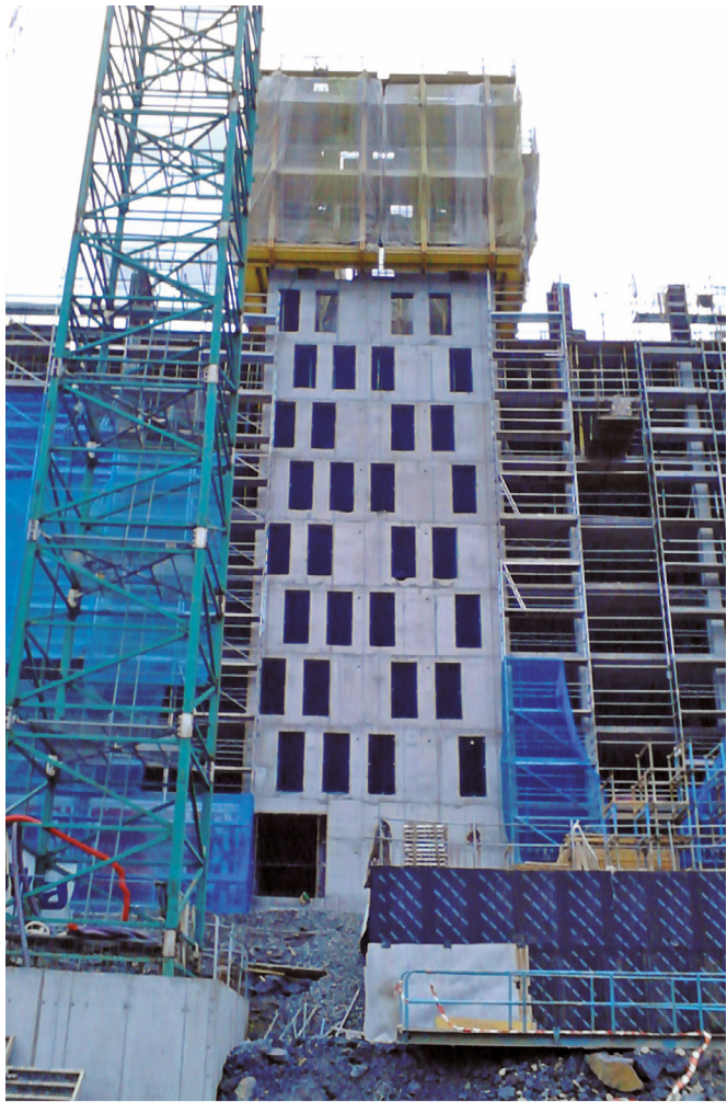
► Roll-back or tilt-back systems to climb and form building cores and walls
