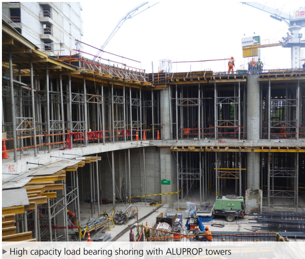
► High capacity load bearing shoring with ALUPROP towers
