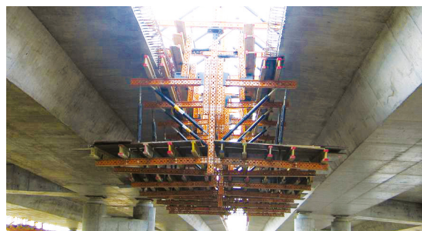
► Parapet form carrier for use on deck edges and between two decks
