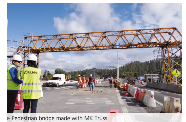
► Reinforced trusses for large span between supports
