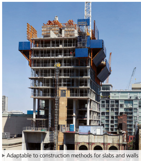
► Exterior formwork and platforms hung from the MK structure above
