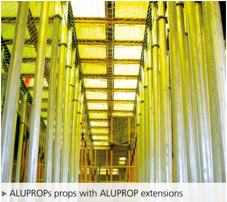
► ALUPROPs props with ALUPROP extensions
