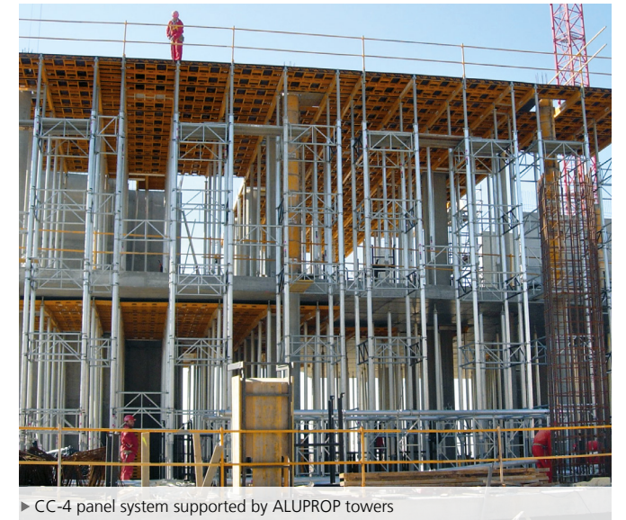
► Change of formwork direction optimizes its layout and reduces infillings
