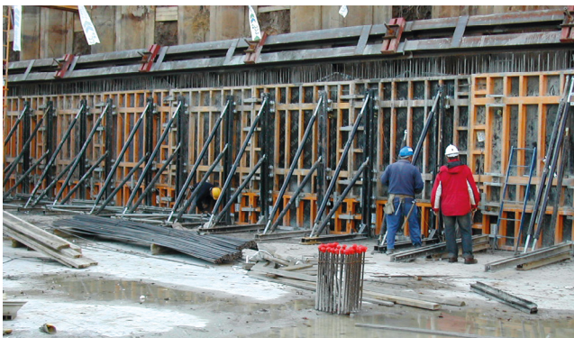
► UCAB frames with MEGAFORM modular formwork
