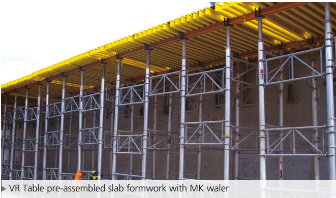
► VR Table pre-assembled slab formwork with H20 wood beam
