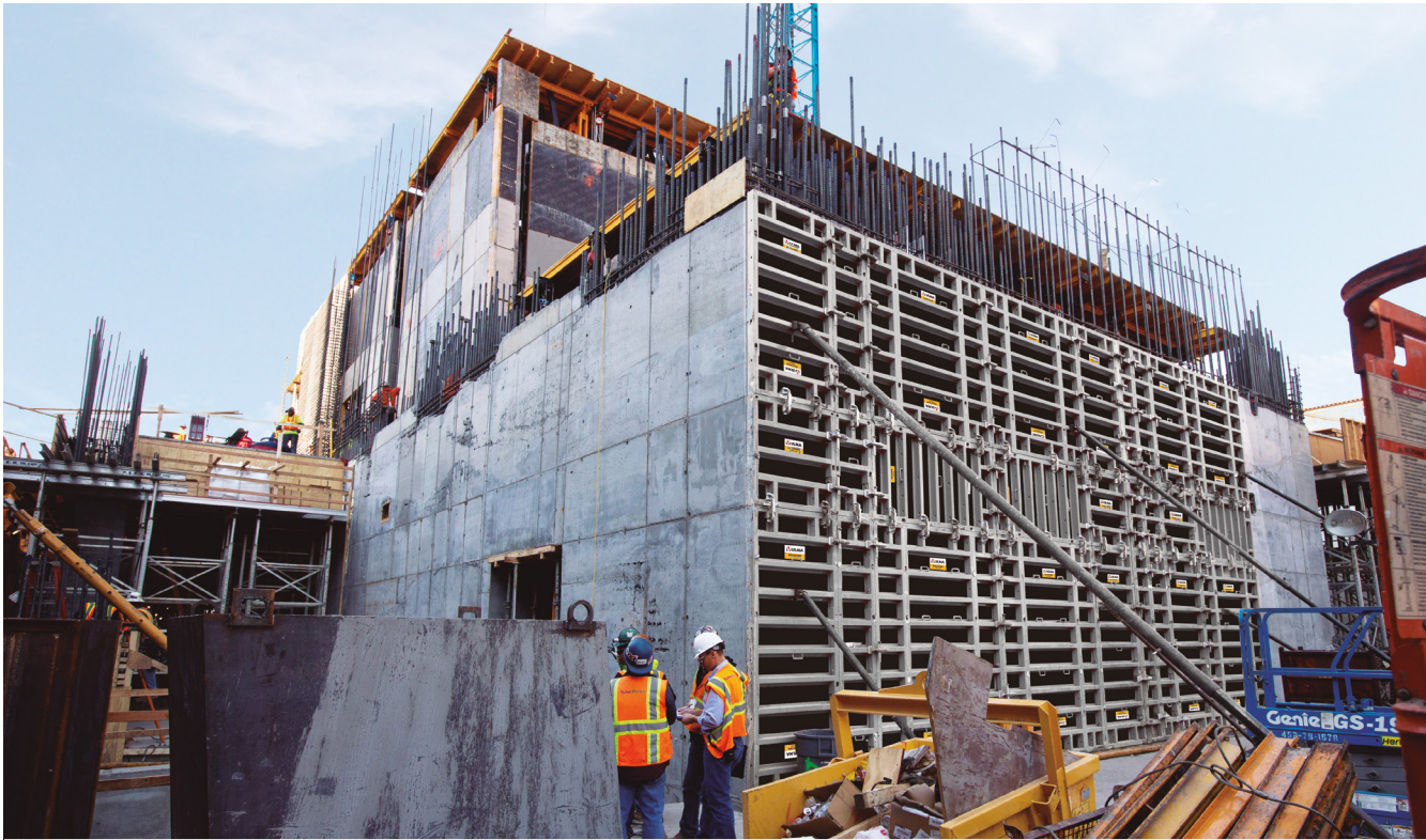
► Indentations in the panel to ease stripping and assist with panel placement
