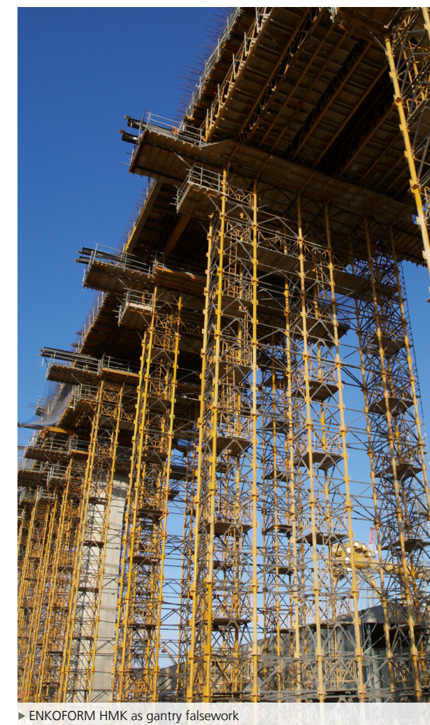
► ENKOFORM HMK as gantry falsework
