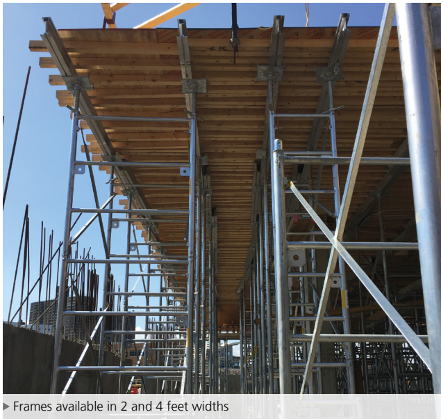
► Two Tie-off plates are located on each frame
