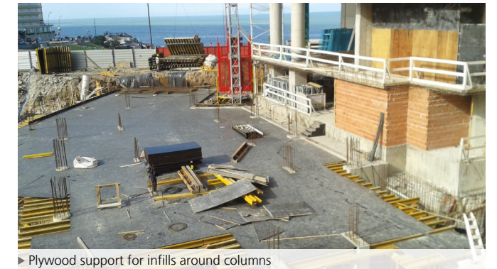
► Plywood support for infills around columns
