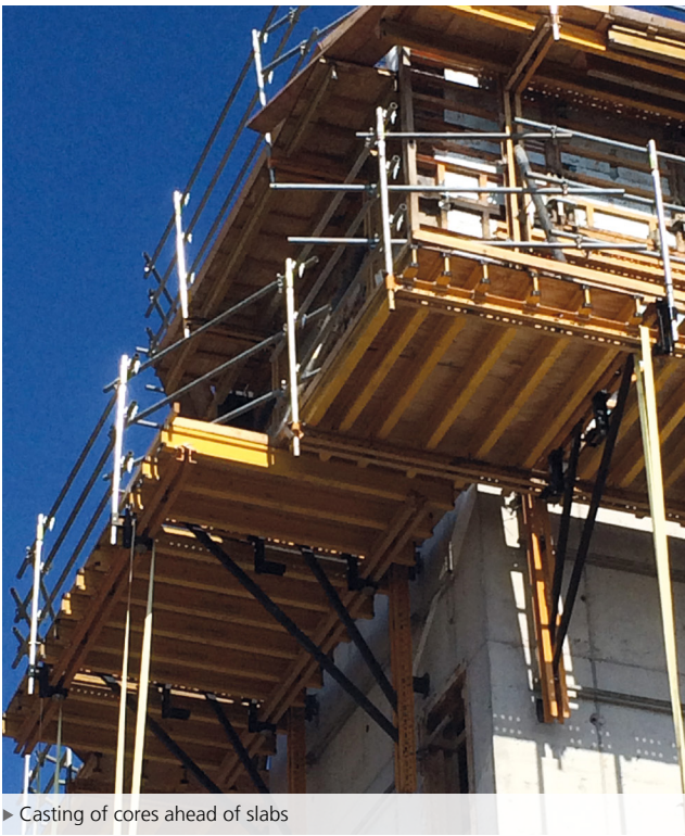
► Casting of cores ahead of slabs
