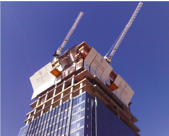
Debris section: slab extension for use as perimeter working platform and material storage area. Prevents debris from falling during formwork table removal and provides a large advertising area directed toward the street below.
