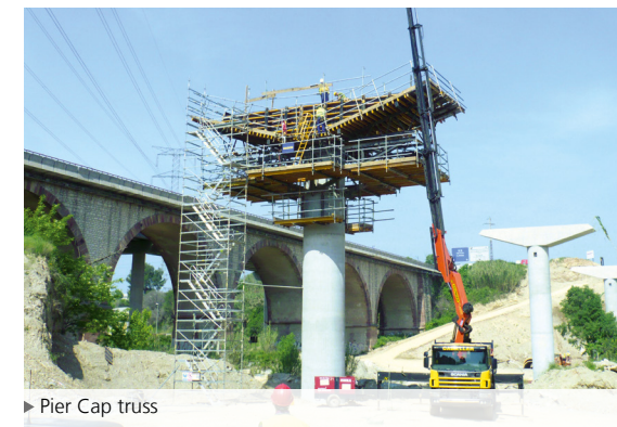
► MK Truss used for gantry falsework
