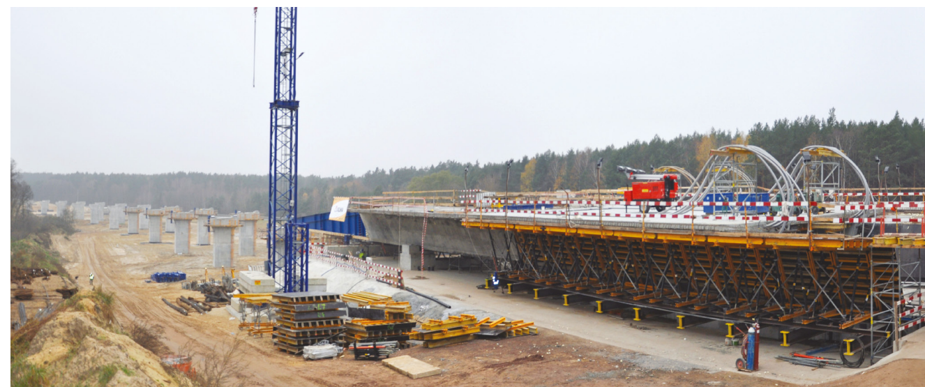
► Incremental bridge construction using ENKOFORM HMK
