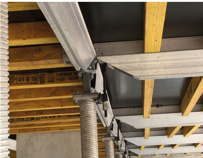
► Hold down brackets for cantilever conditions
