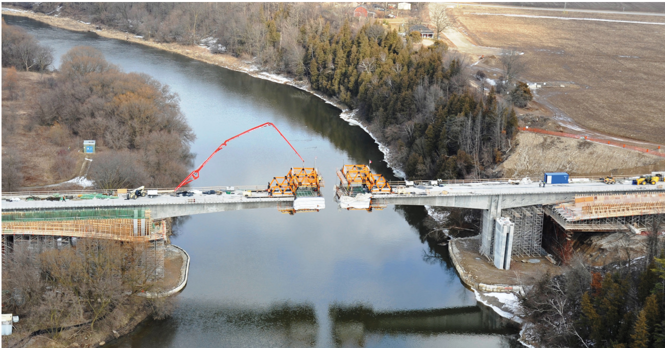
Mobile cantilever formwork carriage for bridge construction.
