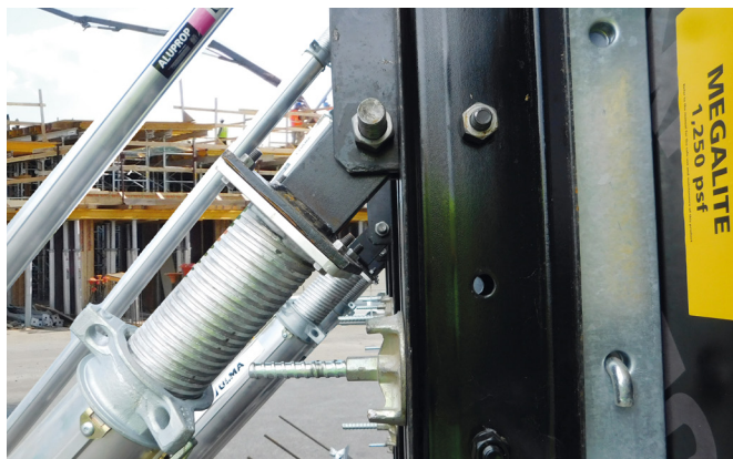
► ALUPROP connection to panel formwork
