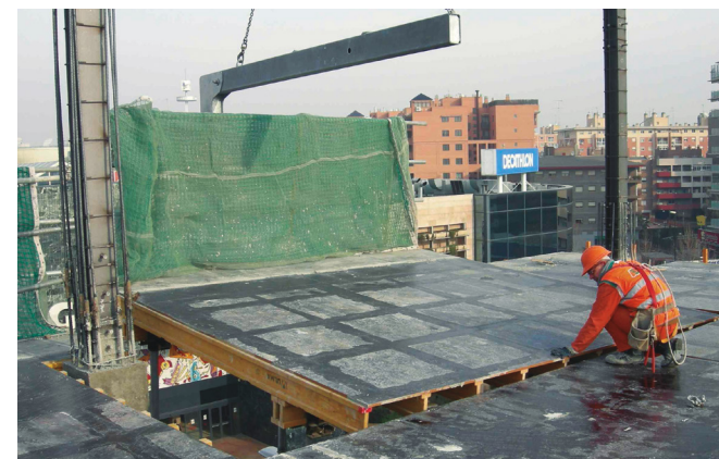
► Lifting and installation of tables with attached handrails
