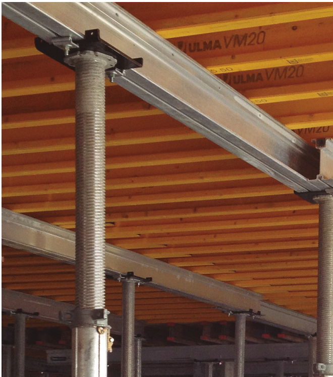
► Aluminum stringer supported by Universal Stringer Head and Stringer clip
