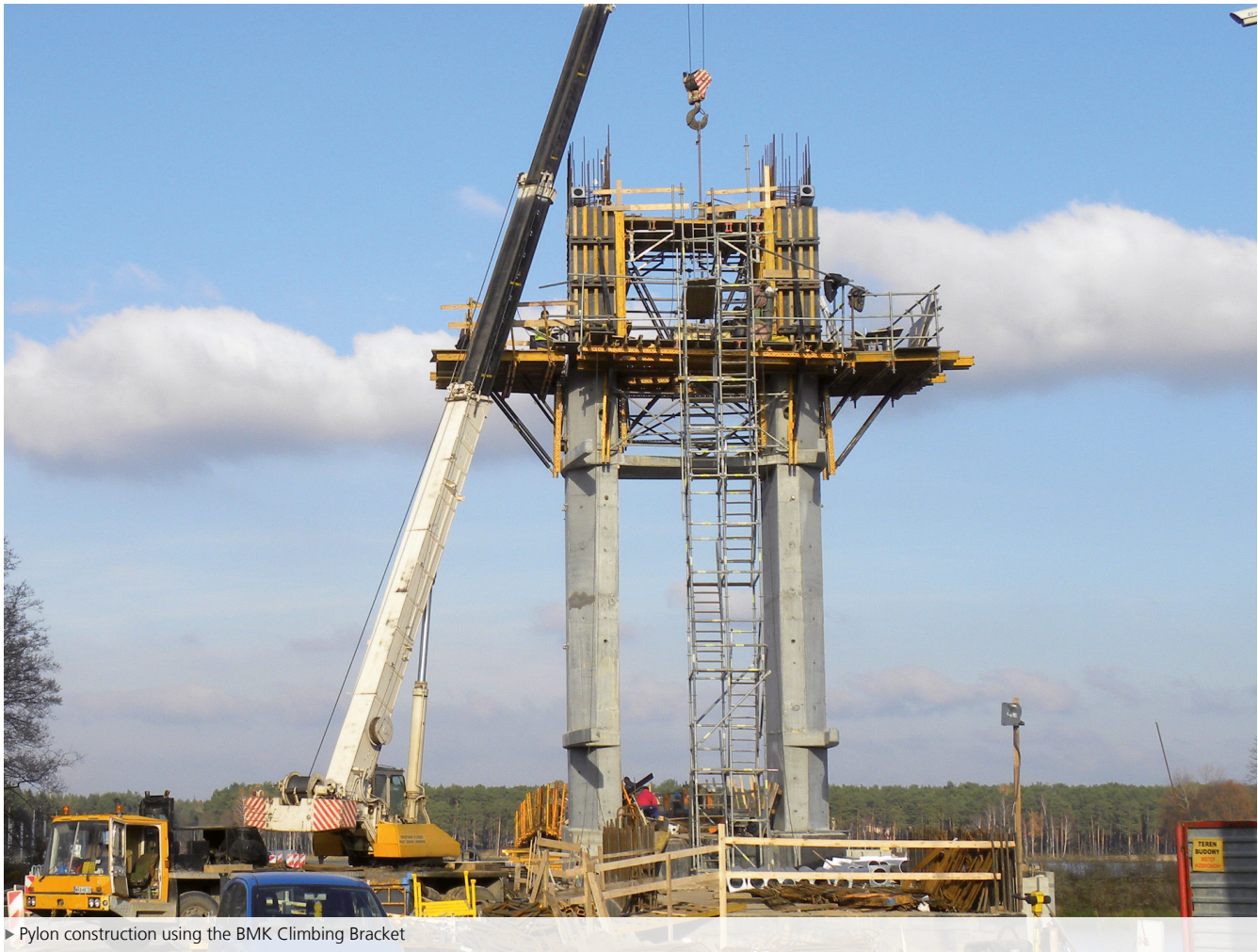
Pylon construction using the BMK Climbing Bracket
