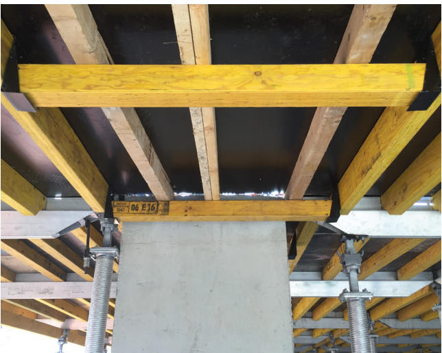
► Infilling around columns
