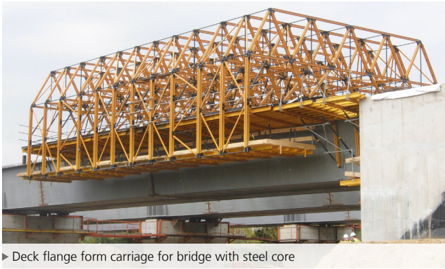
► Deck flange form carriage for bridge with steel core
